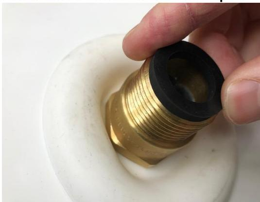
**Connect Stiebel brass adaptor. Fitt off remaining plumbing fittings then Nip up Brass nut**
