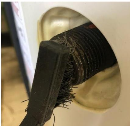
Prepare glass enamel surface with Emery tape or Sand Paper. Ensure glass enamel (the internal pipe) is sanded at least 20 mm past bare metal to ensure Loctite EA3463 adheres/joins to surface.
