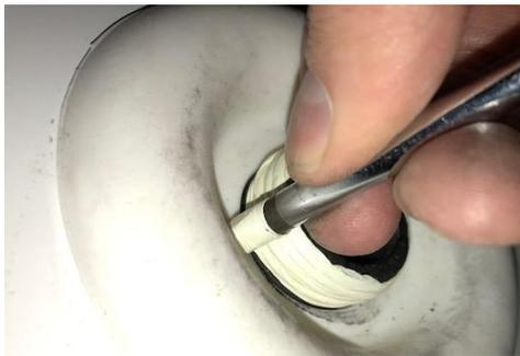
**Ensure edge/face is clear of Teflon so sealing compound can adhere to surface**
