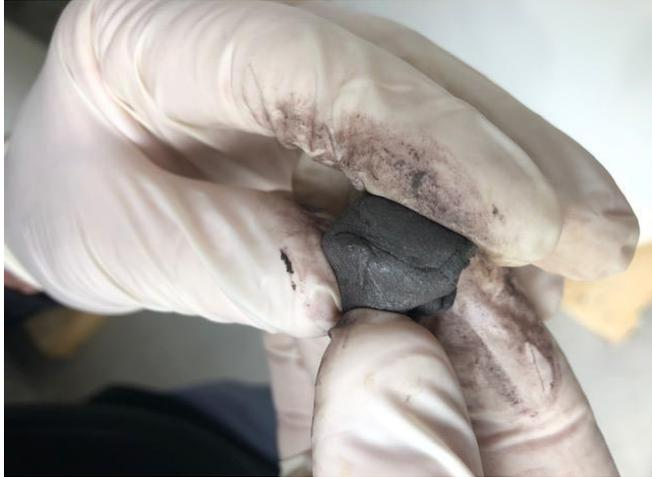
**Apply sealing compound to all prepared metal inside internal diameter surface and 10 mm onto prepared enamel and also 10 mm onto brass surface.**
