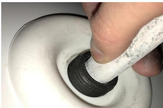
Prepare thread with hack-saw blade or multigrips or other metal tool to enable Teflon to bite into thread
